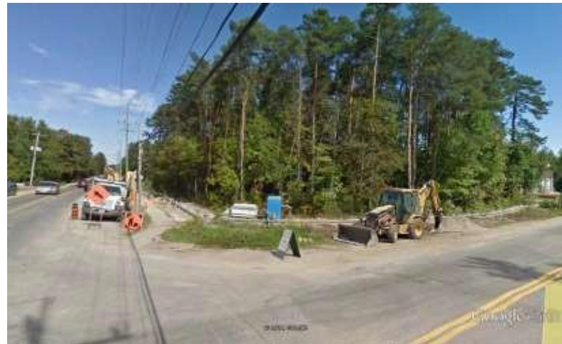
Image 4: Looking northeast at the corner of 25 th Sideroad and Innisfil Beach Road at disturbances caused by road margin-related construction (Imagery date: Sept. 2009).
