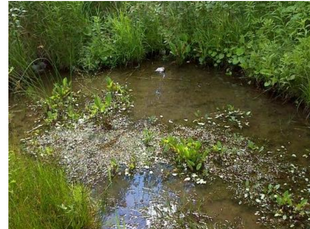
Photo 10: Standing water in overflow channel.
