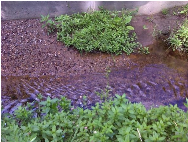
Photo 11: Alcona Creek as it flows out of culvert crossing of 25 th Sideroad.
