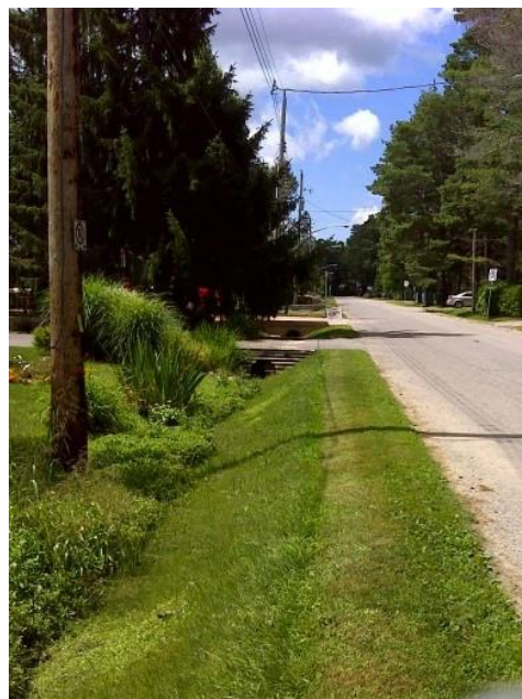
Photo 4: Roadside ditch along Park Road conveys seasonal flow toward Innisfil beach. Standing water in portions of ditch at the time of survey (July 24, 2014).
