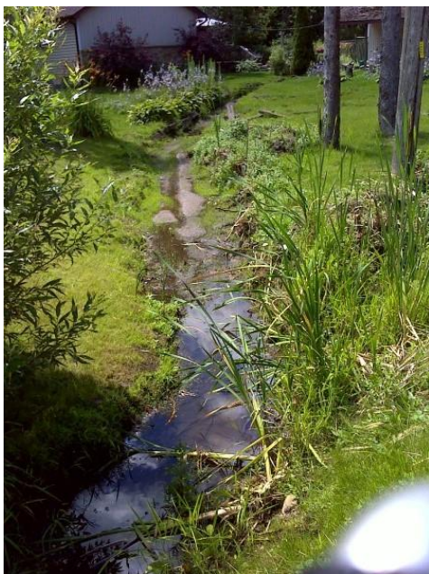
Photo 3: Flow from CUP3-3/FOD3 community is received by channel that cuts through residential properties to Park Road ditch. Dry in upper portion and standing water in channel nearest road (July 24, 2014).
