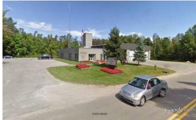
Image 6: Looking northeast along Innisfil Beach Road at existing Fire Hall building, manicured grass lawns, and surrounding undisturbed wooded area. (Imagery date: Sept. 2009).
