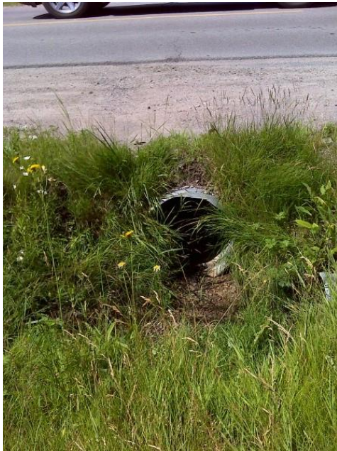
Photo 1: Culvert conveying roadside drainage across 25 Side Road to the CUP3-3/FOD3 community to the east .
